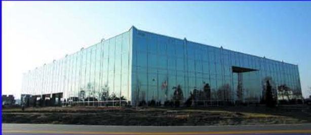
Southern Star Central Gas Pipeline 4700 Highway 56, Owensboro, KY
