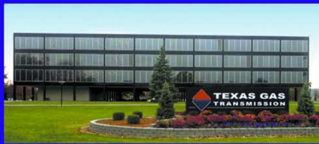
Texas Gas Transmission LLC 3800 Frederica Street, Owensboro, KY
